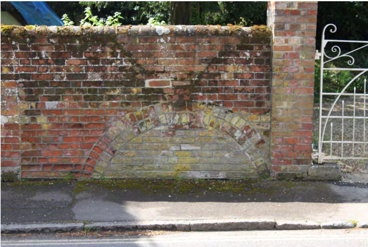
Picture 1.17 Brick archway feature in wall at Cleeve Hall
