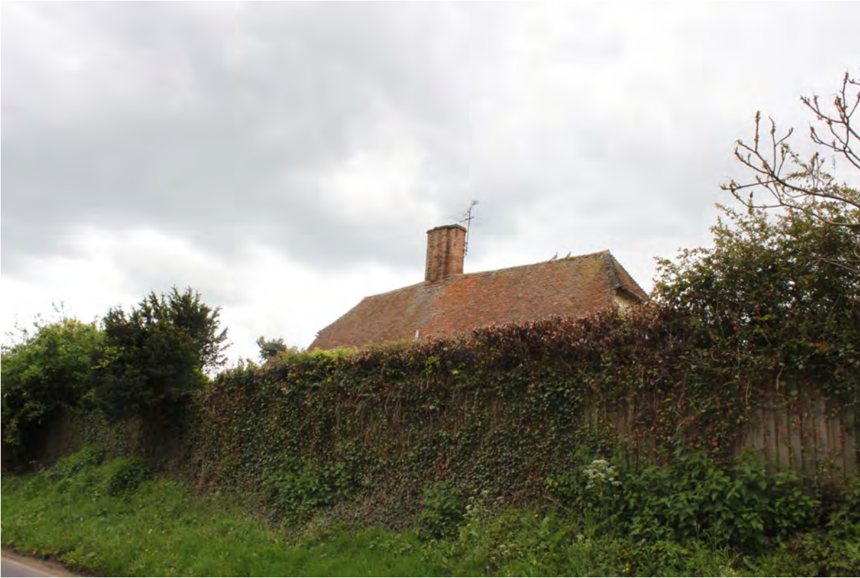
Picture 1.31 Roof of Hill House, Carter Hill
